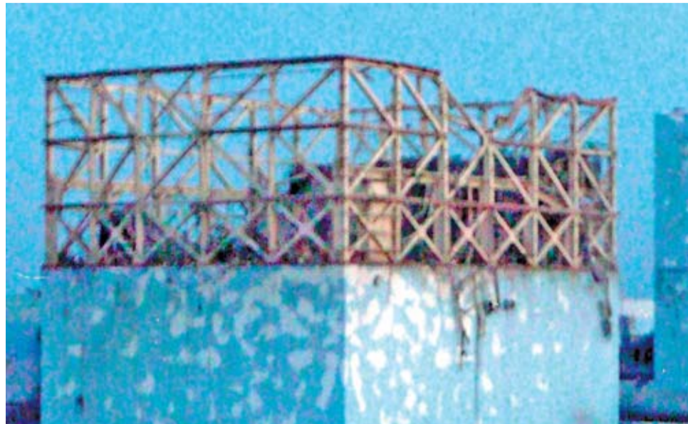
The damaged roof of reactor No. 1 at the Fukushima Daiichi nuclear plant after an explosion that blew off the upper part of the structure.
